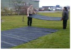
The panels weigh 33 Kgs and can easily be handled by two men. No special tools or equipment are needed.
